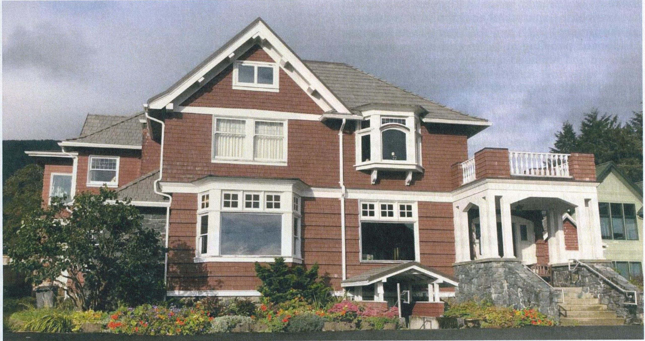
Figure 8.9: Synthetic (plastic) shakes have replaced the original cedar shingle roof.
